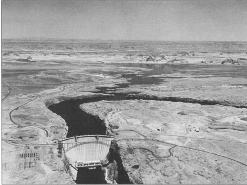
Glen Canyon Dam and Lake Powell, 1966. The dam, composed of 5 million cubic yards of concrete, rises 587 feet from the river bed. The reservoir, the second largest in the United States, can hold 27 million acre feet, about two year's flow of the Colorado. Photo courtesy U. S. Bureau of Reclamation, Regional Office, Salt Lake City, UT.
